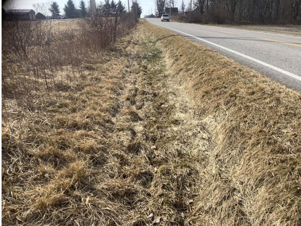
Photo Location 4. View of upland drainage feature. Photograph taken facing south.
